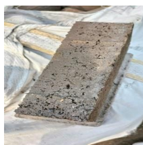
Gambar 4. Defect Geripis (sumber: PT. Pesona Arnos Beton)
