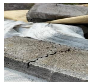
Gambar 5. Defect Retak (sumber: PT. Pesona Arnos Beton)
